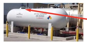
Primary Tank RV will typically be located on top of the tank. There may be other RV's in the system.
