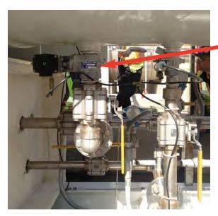
Some valves may be air operated and may even need a signal from a panel to open the valve. It is important to ensure all valves are in the open position.
