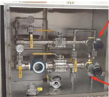
The fill box, pictured here, is a good place to connect the nitrogen bank and the recommend location for pulling vacuum. Use the hose provided and connect to the 1" vapor Epsilon fitting. The other hose end can be fitted with a connection for the nitrogen bank or vacuum pump.
