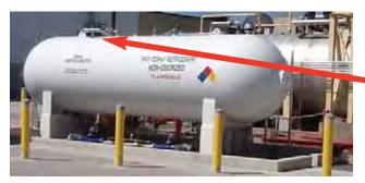
Primary Tank RV will typically be located on top of the tank. There may be other RV's in the system.
