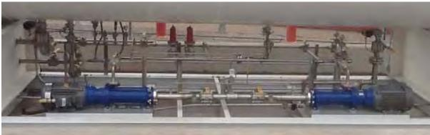
There are a lot of valves on the bottom of the tank to open, be sure to get them all. You can use the pressure gauges to monitor pressures. There should also be bleed points to relieve the pressure during the purge step(s).
