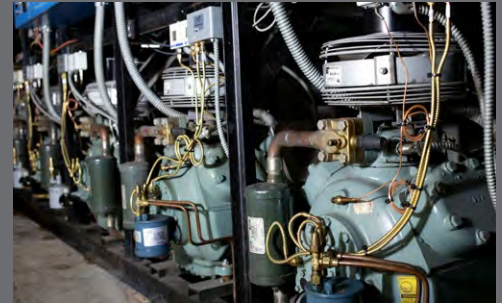
The RRRink’s two parallel compressor racks
