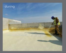
When applied, spray foam creates a seamless, monolithic insulation layer. There are no joints, fasteners and thermal bridges. It is water resistant, durable, and its strong adhesion properties help prevent roof uplift during high winds and extreme weather.
