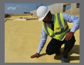
The foam is carefully checked after it hardens to ensure that the installation meets high quality standards.
