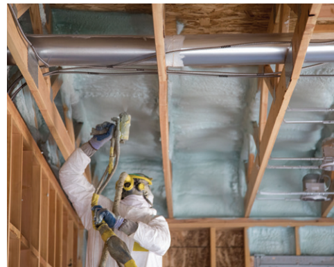
While spraying overhead, the foam demonstrated excellent adhesion which reduced dripping.
