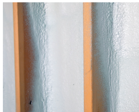
Demilec's new wall foam provided an exceptionally smooth surface finish.
