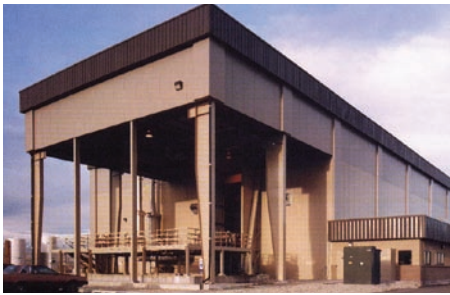
Salt Lake City Sodium-Reduced Sponge Facility
