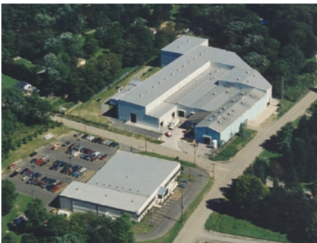
Fombell, Pennsylvania Facility
