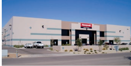
Honeywell's electronic chemicals manufacturing site in Chandler, Arizona.
